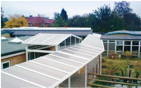
Free-standing Covered Walkway
