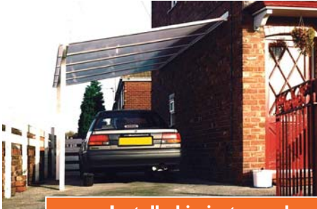
Installed in just one day
