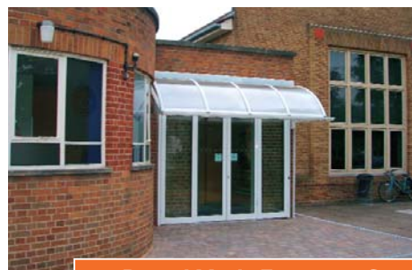
Barrel Vault Entrance Canopy
