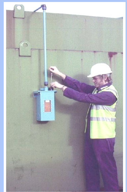
Wall mounted 610 Tank Vent Dryer
