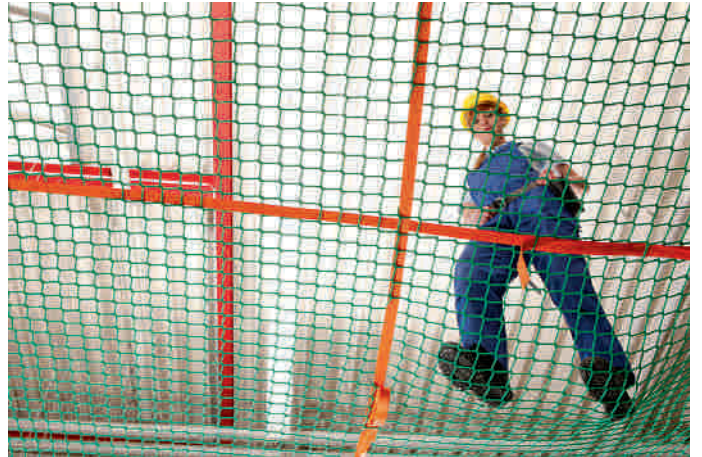
Page 21 Safety Nets as Work Platforms
