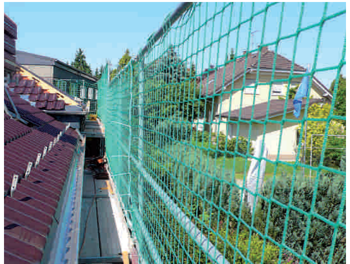
The guardrail is secured to the load-bearing construction mesh.
