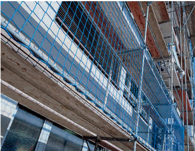
The guardrail is secured to the load-bearing construction mesh.
