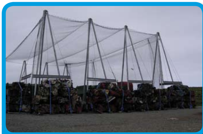
Western Isles Council - HDT Enclosure
