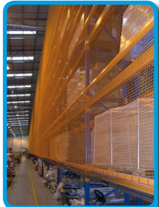
Factory Pallet Rack Netting
