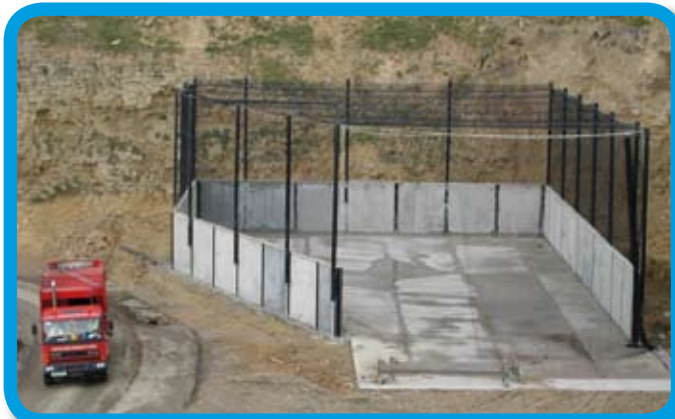
Houghton-Le-Spring - Storage Bay
