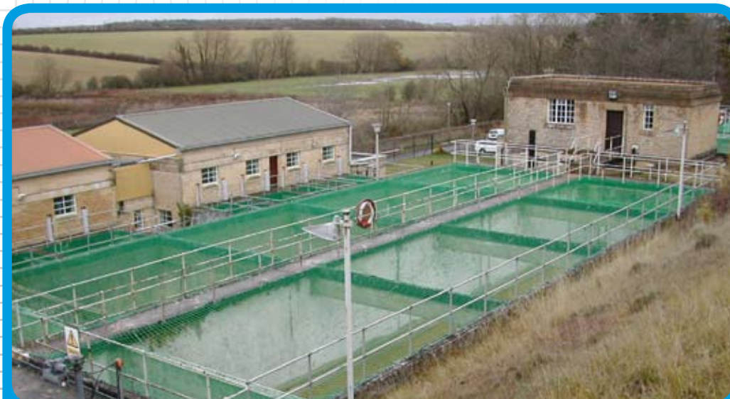
Tank - Catch Netting
