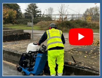
Sawing with Bycon DFS500 Petrol Floor Saw
