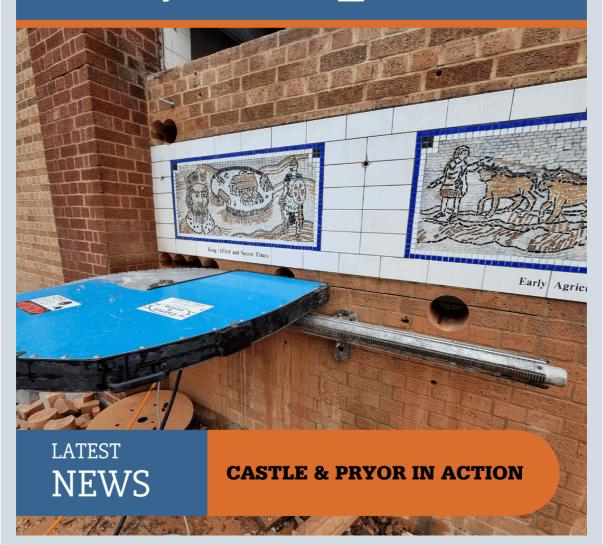
In preparation for the demolition of Farnborough Leisure Centre in 2022, a freeze of 16 murals needed to be removed in order to preserve them for the future. This is where our track sawing and diamond drilling expertise came in to help.
