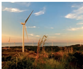
Burgos Wind Farm Project - Philippines
