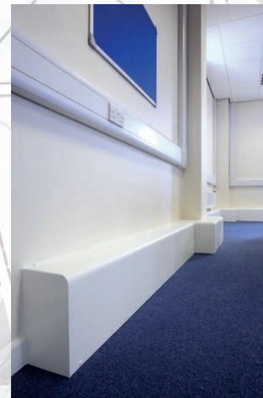
VERSA 8 PRE-FORMED PLYWOOD CASING HEATING REFURB, NHS TRUST, DARLINGTON
