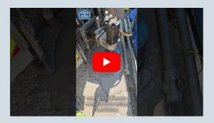
Using our trailer rig we Diamond Drilled 30nr 182mm diameter holes for bollard installation.
