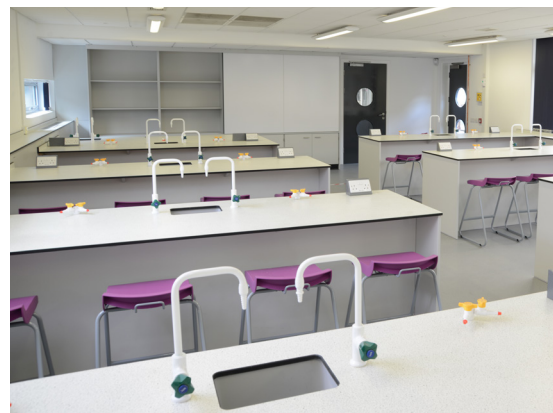
Slough & Eton C of E College FULL REFURBISHMENT OF 6 SCIENCE LABS & PREP
