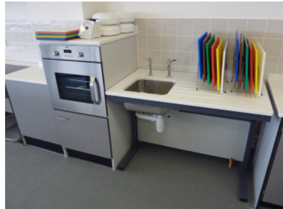
Mid height oven and adjustable height sink unit
