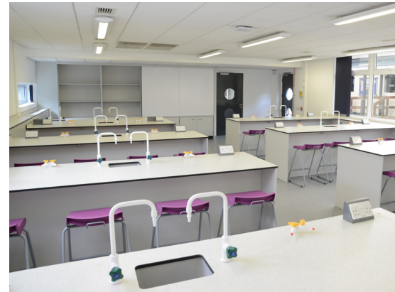
Trespa benching mounted with gas, electric outlets & sinks
