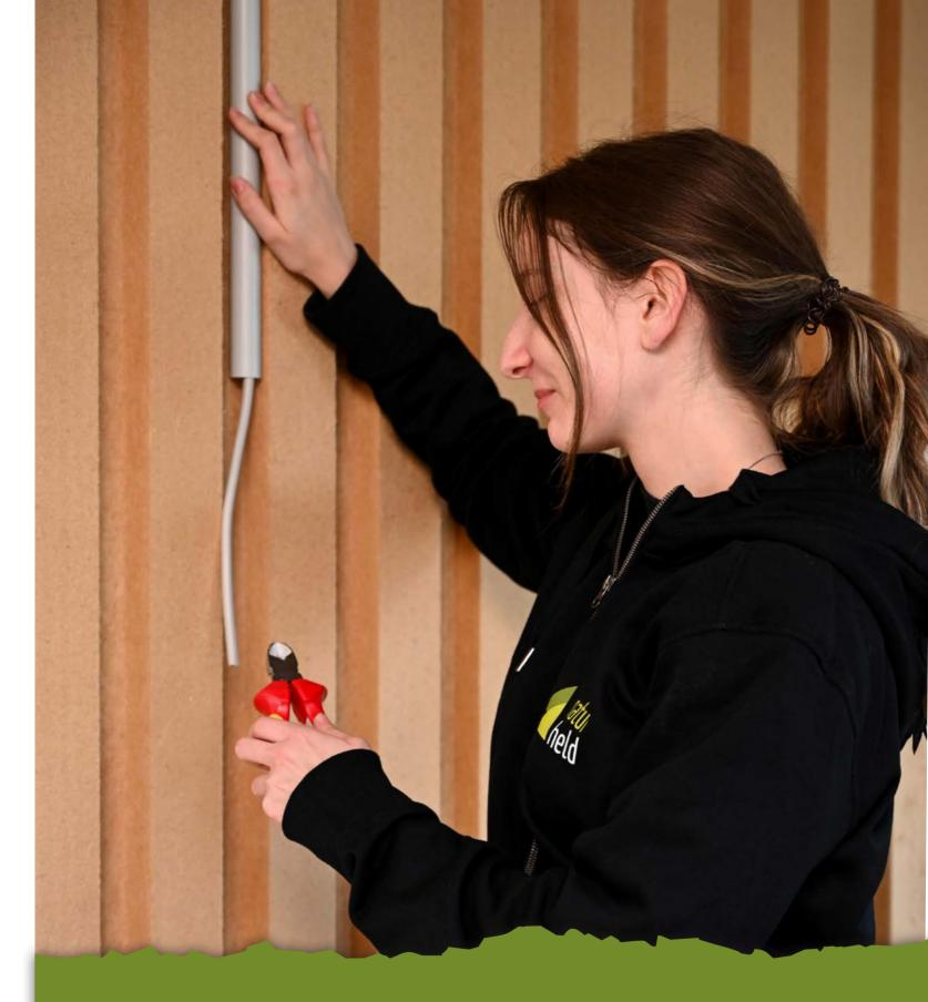
With naturheld 140-Install, installers can reduce installation time on site. The solid wood fibre insulation board is factory-fitted with pre-milled installation channels.
