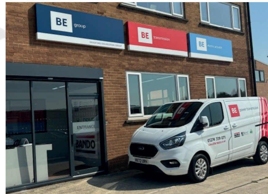
BE Power Transmission, Head Office and Trade Counter, Bradford.
