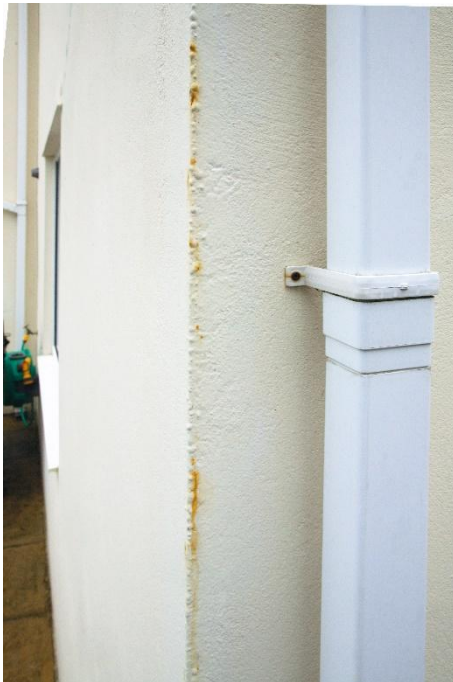
Image 2: Examples of building render where steel render beads have been used, which has led to rust leaking into the render, causing unpleasant discolouration and damage
