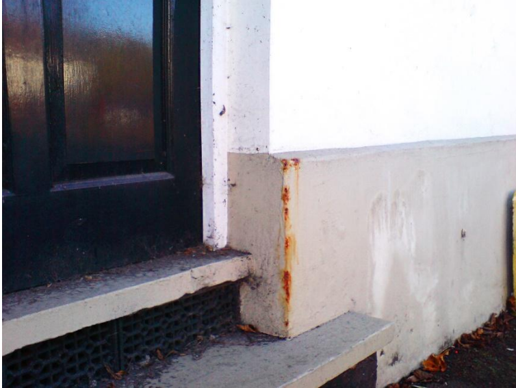
Image 3: Examples of building render where steel render beads have been used, which has led to rust leaking into the render, causing unpleasant discolouration and damage
