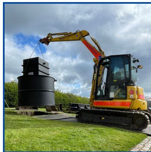
Systems easy to offload and handle on-site
