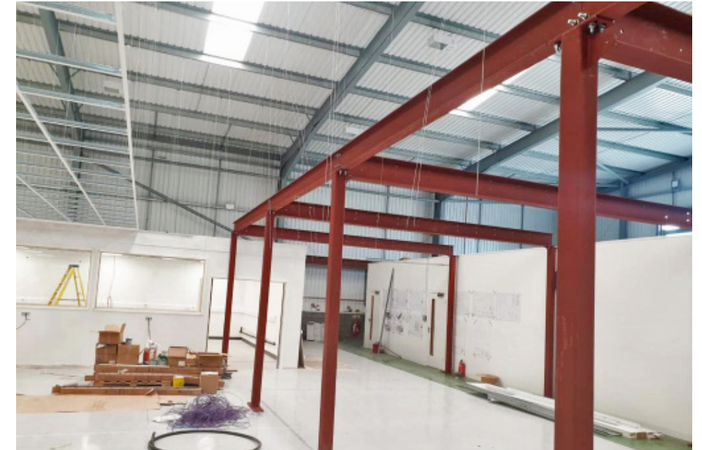
Steel support for mezzanine
