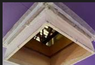
Ply box Loft hatch
