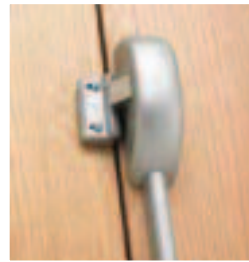
Upper side Pullman latch (shown on double door application)
