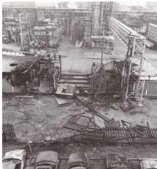
Figure 1 During cleaning of residue from a distillation vessel used to recover an aromatic nitro compound, an incandescent flame erupted from the vessel scorching a path through a nearby building before hitting a large office block. Two employees were killed instantly and three others, including a young office worker, died from their injuries several days after the incident. The company was prosecuted for an alleged breach of section 2(1) of the Health and Safety at Work etc Act 1974 and fined £250 000, with costs of £150 000 awarded to HSE
