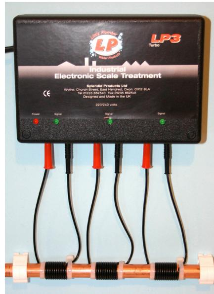
In March 2002 Hospital Metalcraft installed 2 x LP3 units to remove and prevent limescale which was causing a problem to their equipment. The problem was such that production was being affected because the water was so hard and limescale was affecting the finishing processes.
