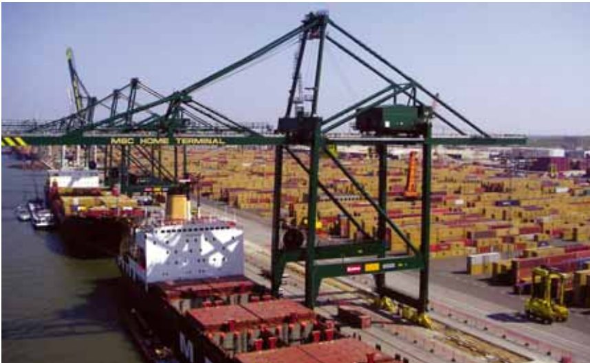
STS cranes in Antwerp with igus® Energy Chain Systems® for energy and data supplies to centenary and main trolley.
