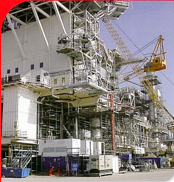
12.5MVA Loadtest on the W.A Platform in Baku
