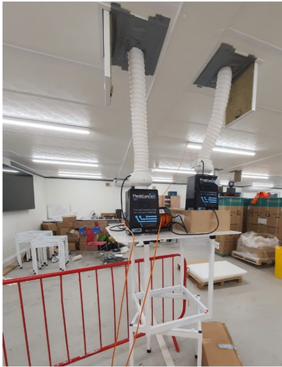
Dry micro-misting SMS at positive pressure
