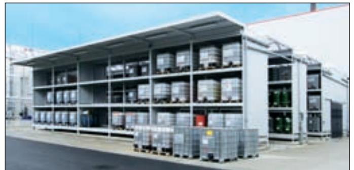
Large storage facility for about 400 tonnes of hazardous material in drums, IBC/ASF and further special containers, completely roofed, with efficient accessibility to all containers.
