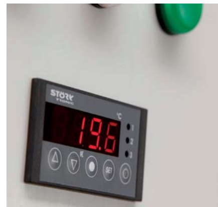
Temperature controller (thermostat)
