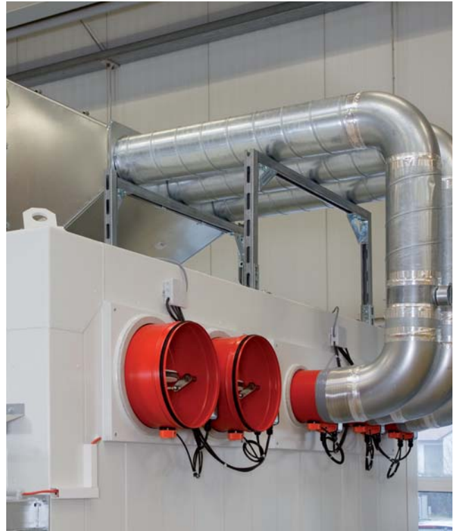
Inlet and outlet air connections with fire protection flaps
