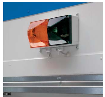
Warning lamp and eaves
