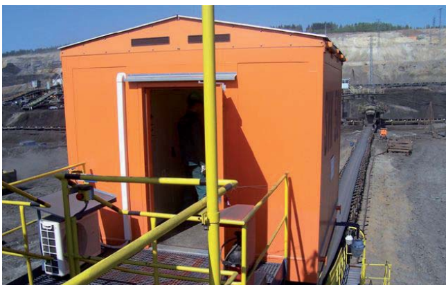
Access to technical rooms
