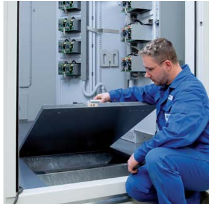
Double floor with door opening
