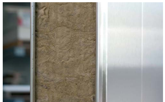
100 mm panels made of rockwool with stainless steel sheeting
