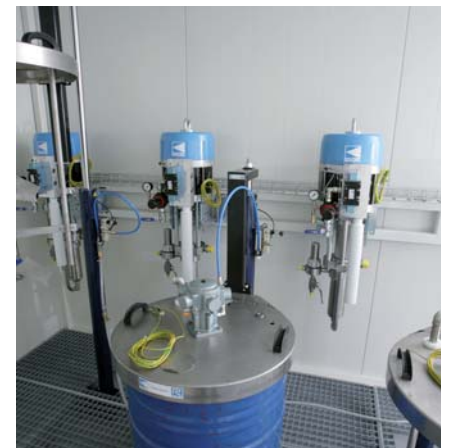
Fixing of fittings/installations in the container
