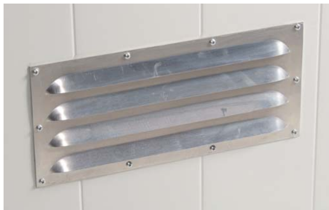
Ventilation component in sidewall with rain protection
