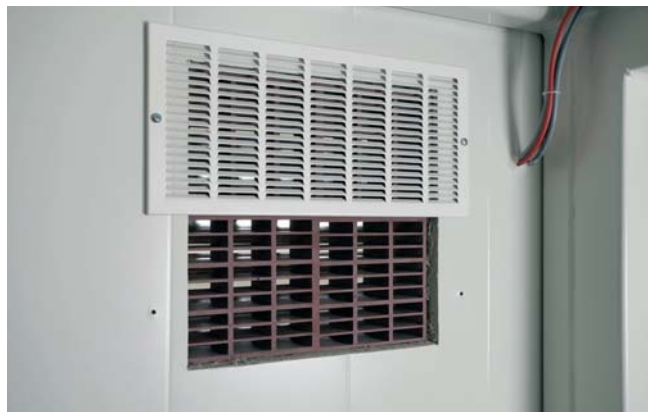
Ventilation component with safety fuse
