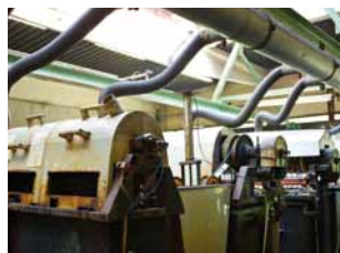
Continuous galvanizing line
