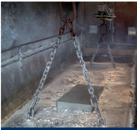
Addition of zinc blocks
