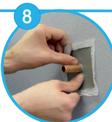
Applying OTL 026 Pipe Sleeve
