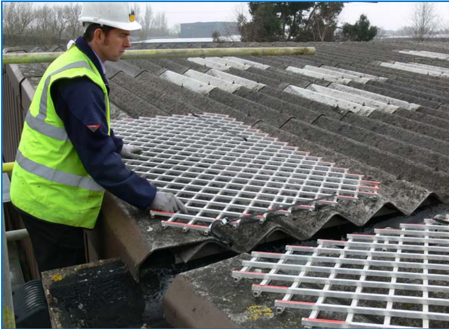
Spreading the first mats each side of a valley where work is to take place
