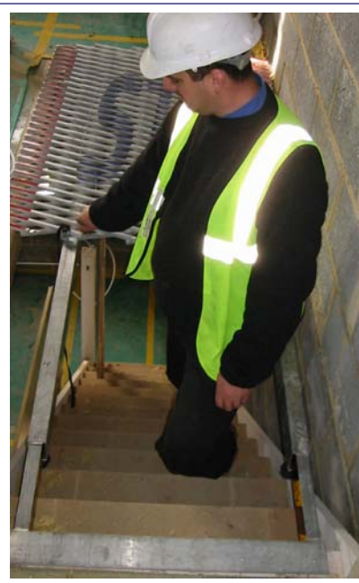
Safe platform for stair void. Keeps full access up stairs or via a ladder before stairs are fitted
