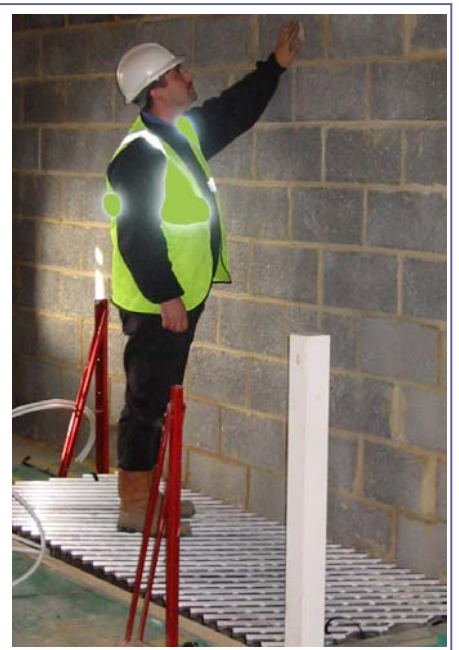
Safe platform for stair void. Keeps full access up stairs or via a ladder before stairs are fitted
