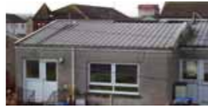
Roofing prior to refurbishment
