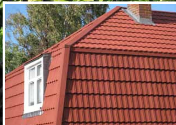
Complex ridge detailing using Metrotile barges & end cap accessories
