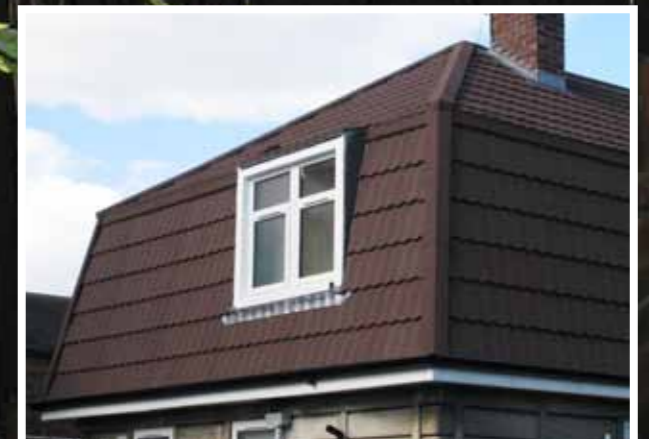
A refurbished roof in Bronze Bond
