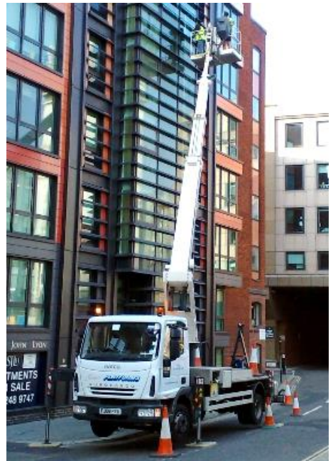
Below, The LM22 reaches from the road side
