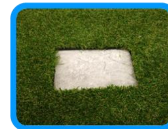
Place tape under repair
