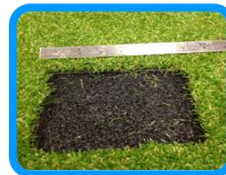
Cut back damaged turf
