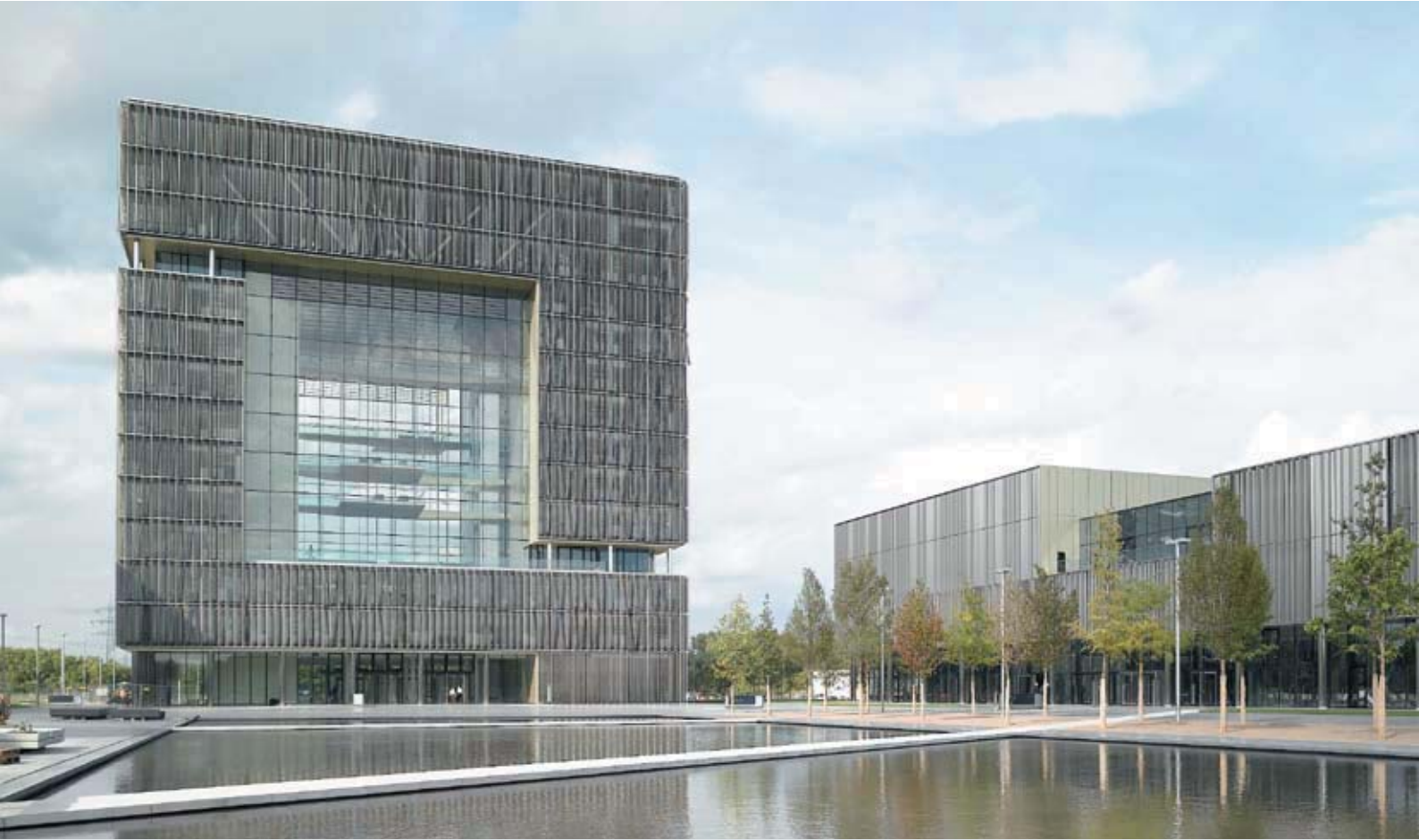
ThyssenKrupp Quartier in Essen with Hörmann products
