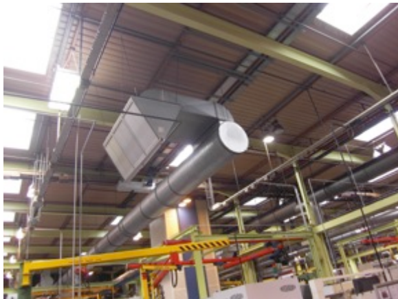
X-CYCLONE® air cleaner in a German gear production factory in Baden-Württemberg
