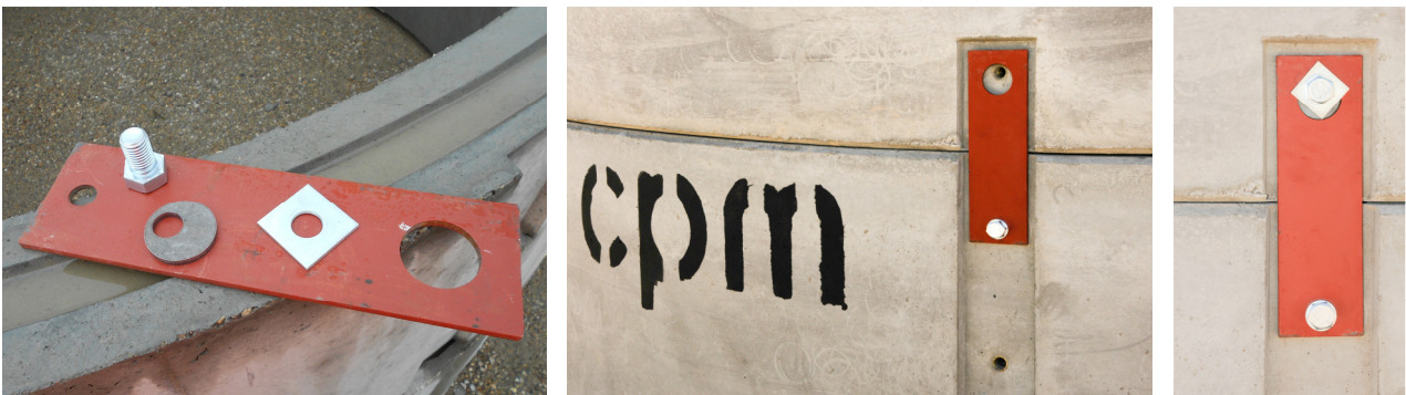
Fig A2 - Joint Connecting Plate
