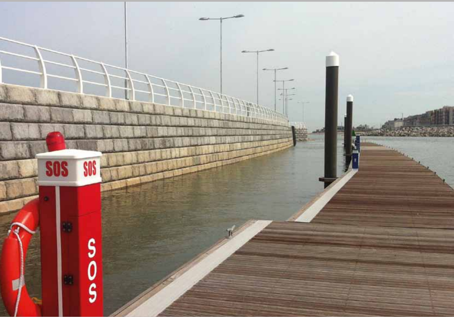
Rhyl Harbour Quay Wall, North Wales
