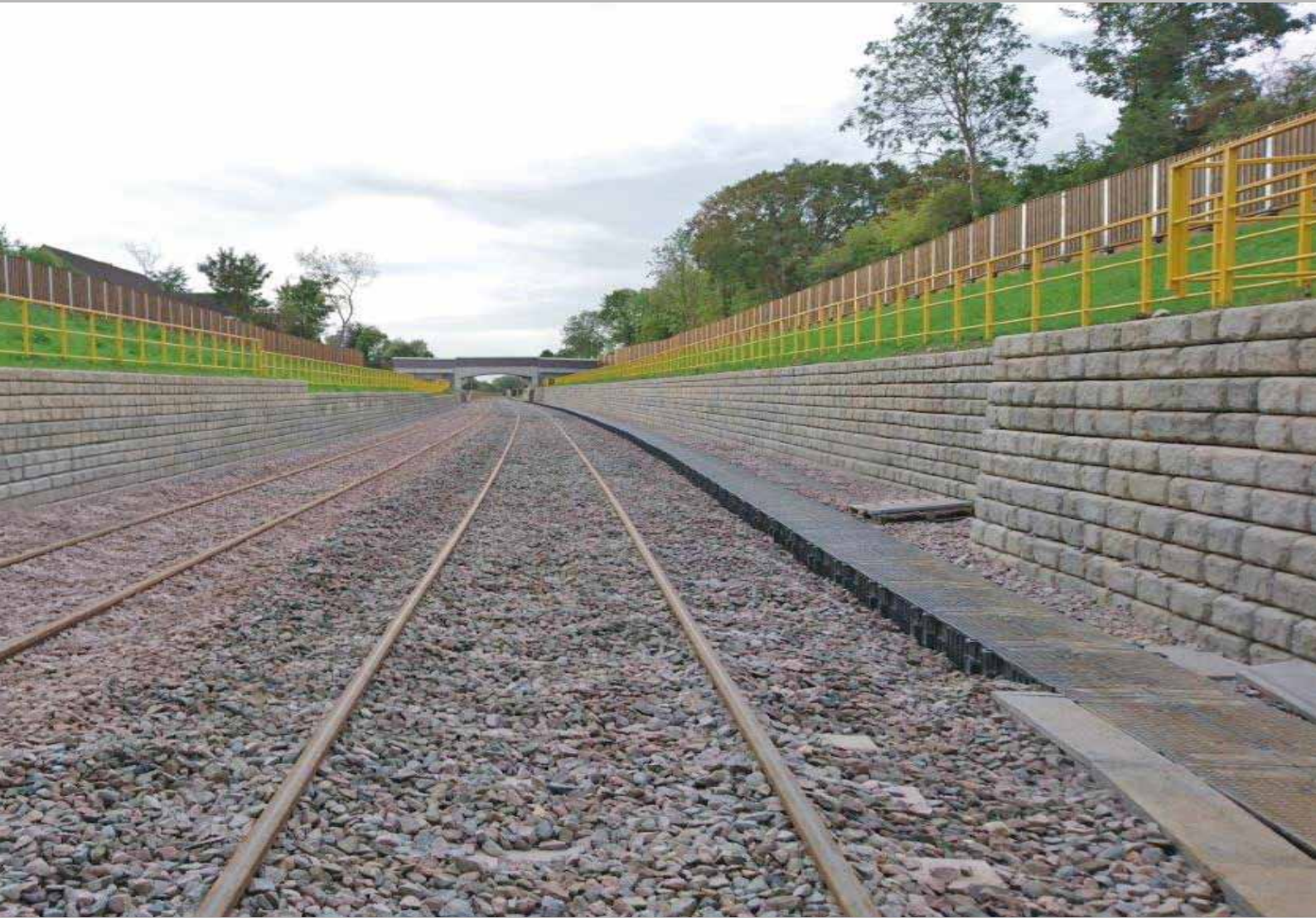
Carillion / Buckingham JV, Bicester to Oxford Route
