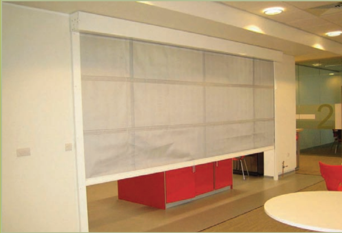
Harling HS Smoke barrier, fire rated curtain partly closed
