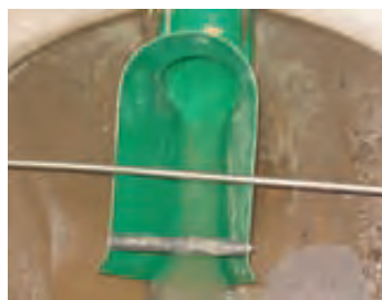
Manhole flume available from DN 100 ( Q_{max} 5,7 l/s) to DN 300 ( Q_{max} 94,4 l/s).
