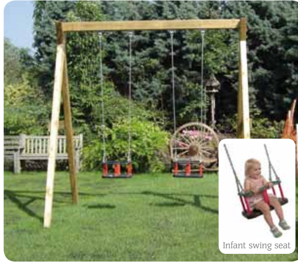
A single bay swing frame with two infant seats newly installed on grassmats.
