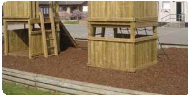
Bark installation with a pair of Jungle Clubhouses.
