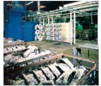
Continuous passage monorail shot blast plant
