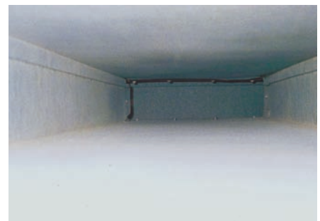
Extract duct after cleaning
