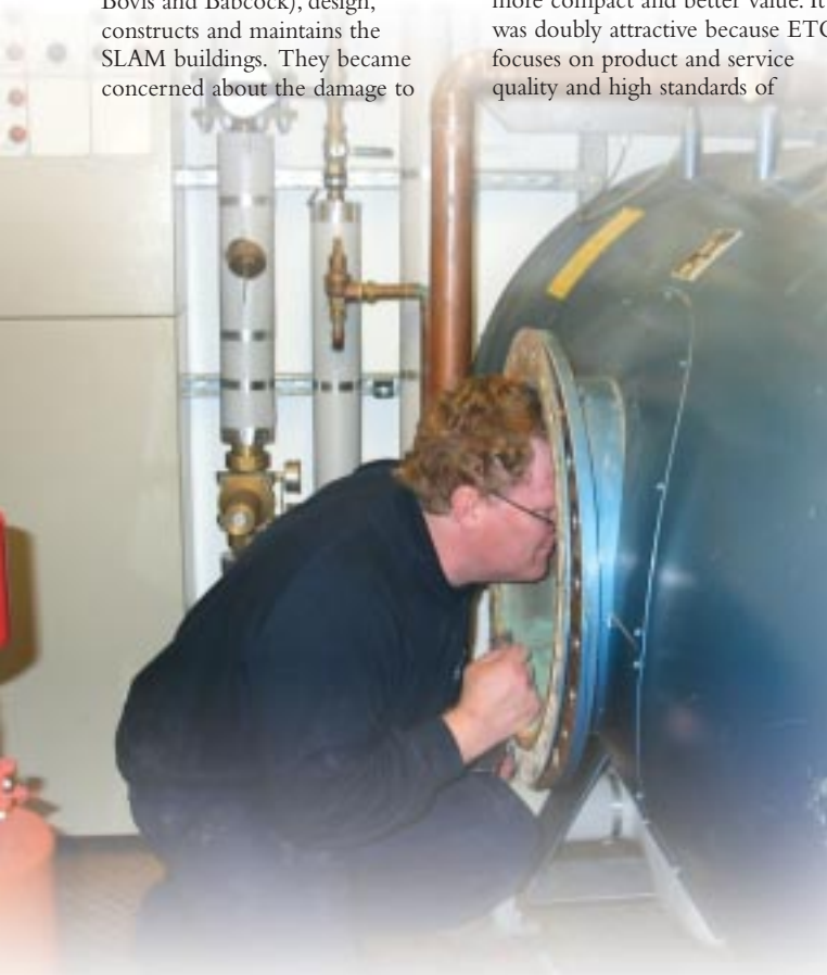
Inspection of the calorifier's heat exchanger
