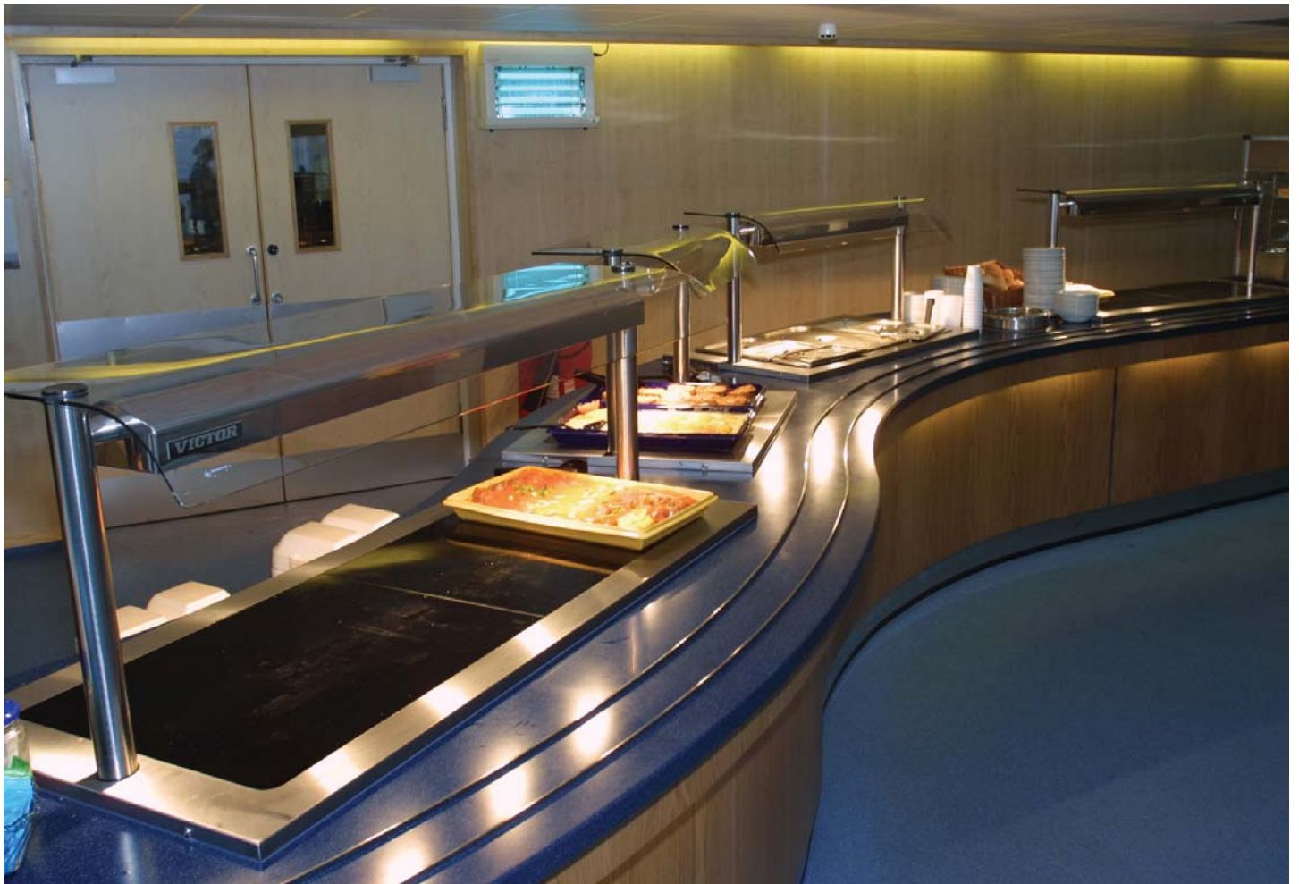
Hospital shop-fitted counter approx. 18 metres long - Corian top with illumination under light pelmet.
