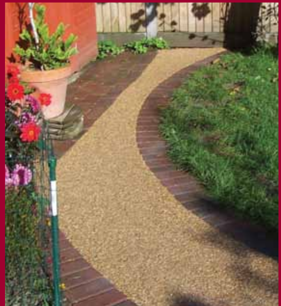
After SureSet permeable paving.
