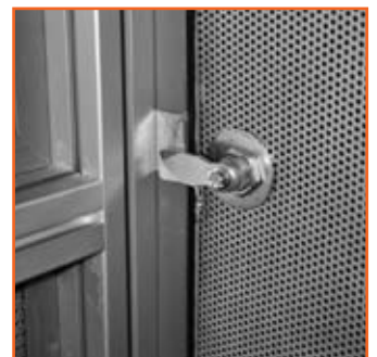
panel fixed with bolt lock
