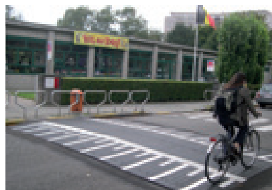
Sinusoidal hump in Gent, Belgium
