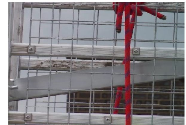
D. Tie a strap or rope to the top rung of the Board-Walk in preparation for lowering it onto the roof
