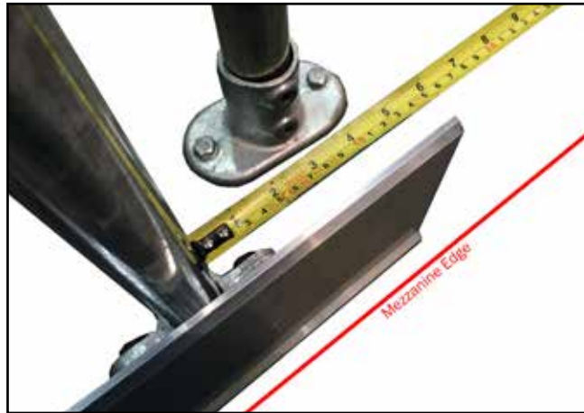
13. Check part (H) toe-board is central within the frame and tighten nuts to 15Nm to ensure it is held securely in place.
